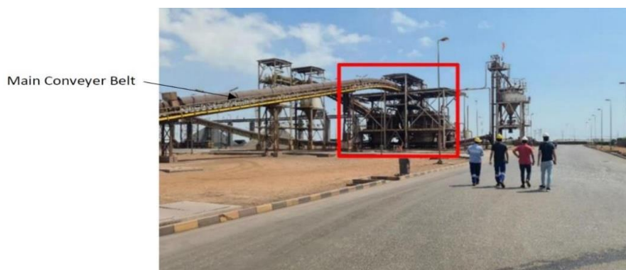
Fig. 2: The screening facility at the steel factory.
